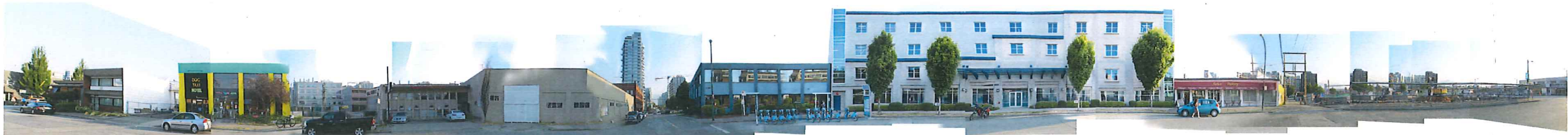
1 East 3rd Avenue looking north
