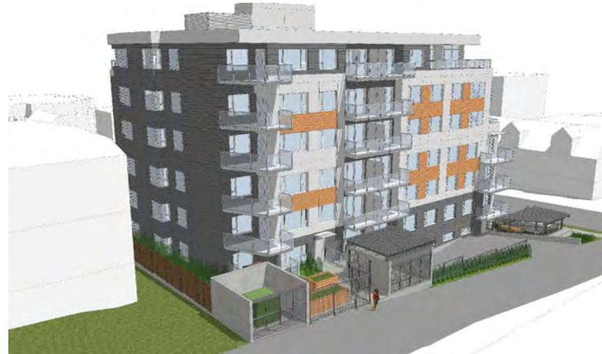
View 2 From lane looking Northeast
