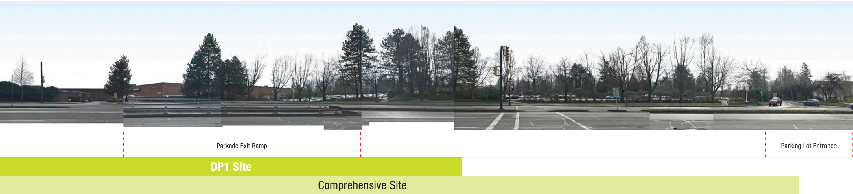
3 West 41st Avenue Looking South
