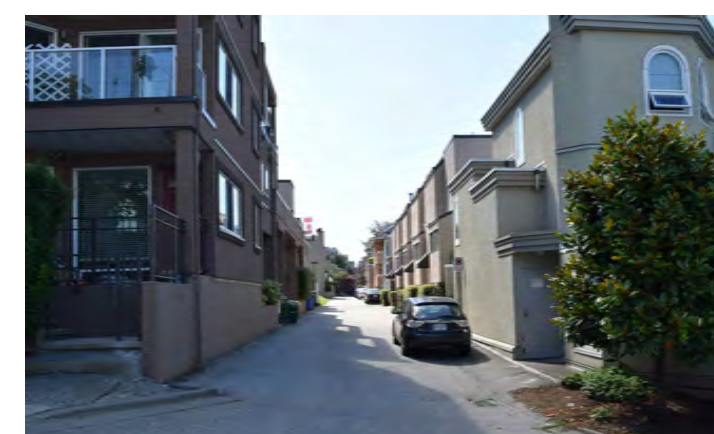
5. LANE VIEW FROM ALDER STREET
