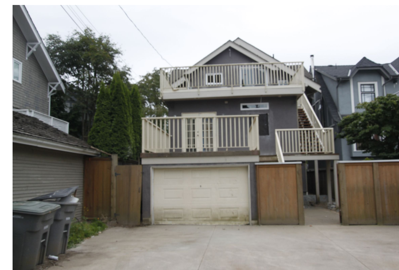
② EXISTING BUILDING (NORTH ELEVATION)
