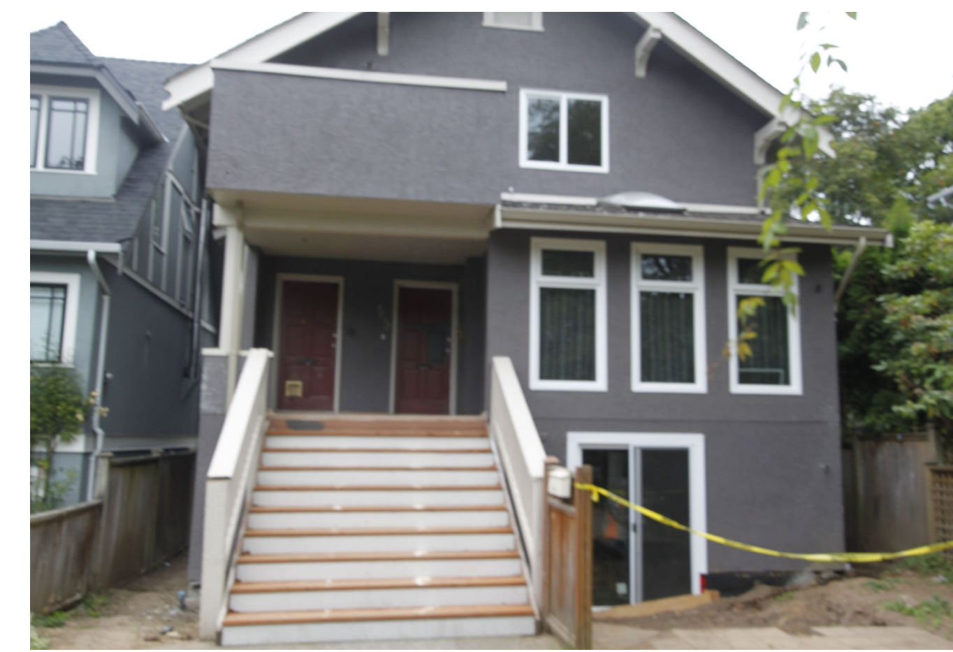
① EXISTING BUILDING (SOUTH ELEVATION)
